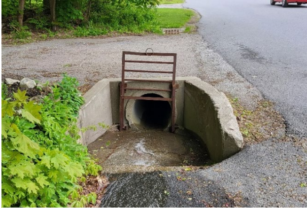
Figure 3: Concrete headwall structure with an 18" drop leading to a 24" RCP inlet to the enclosed system.
