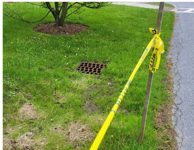
Figure 4: Catch basin inlet at end of Spring Street where recent swale reshaping has taken place.
