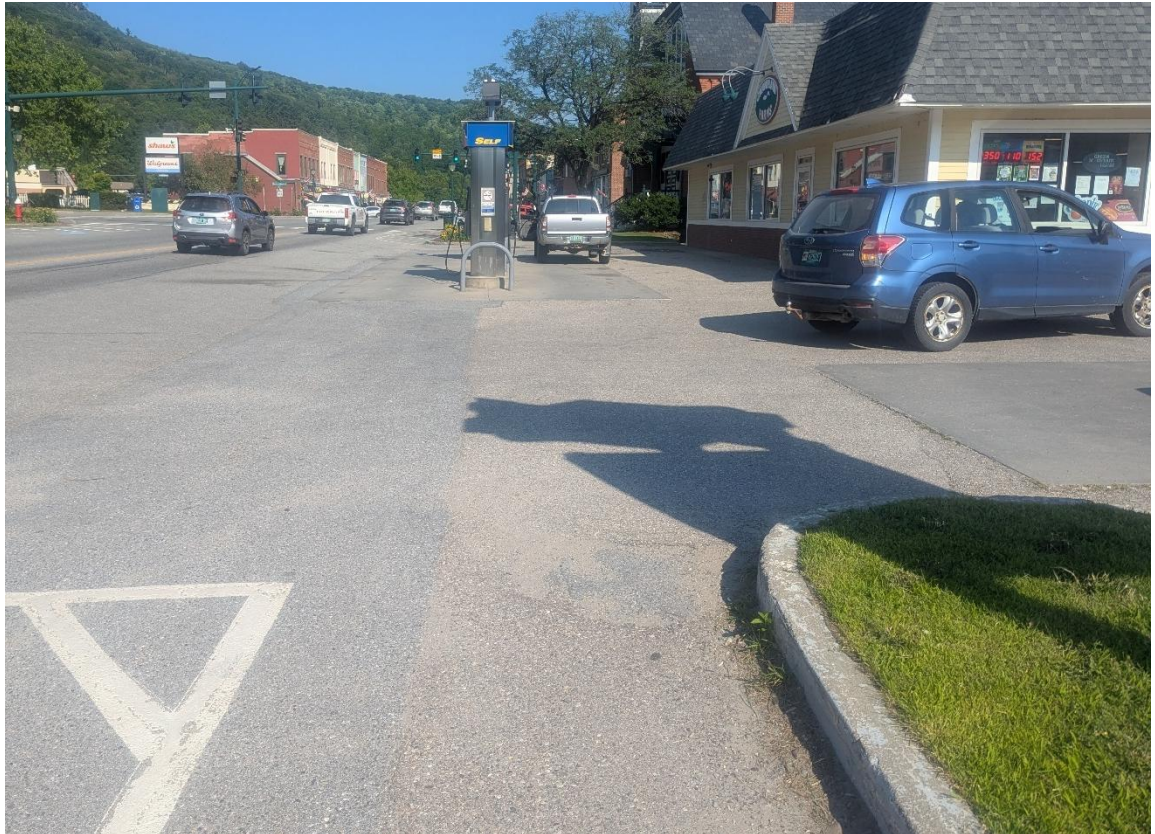
Photo 1 Gap in Sidewalk at Champlain Farms
