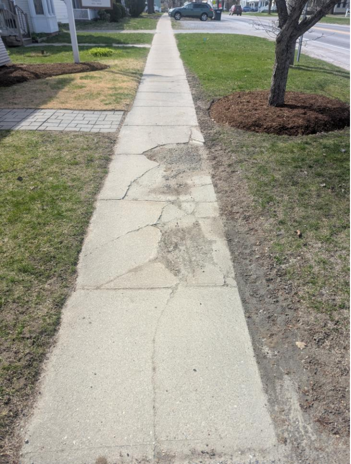
Deteriorated Concrete
