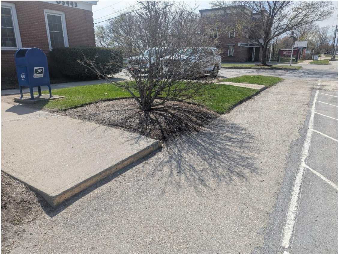
Photo 4 Inaccessible Grade Separation
