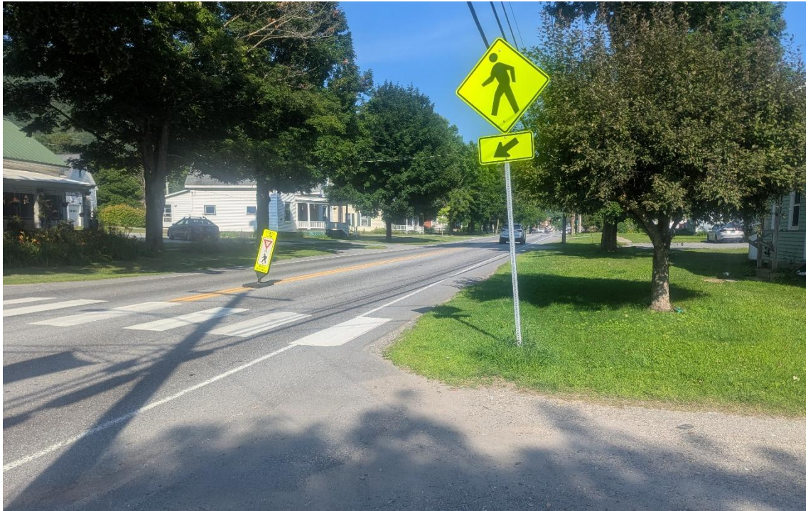
Photo 6 Crosswalk without Landing
