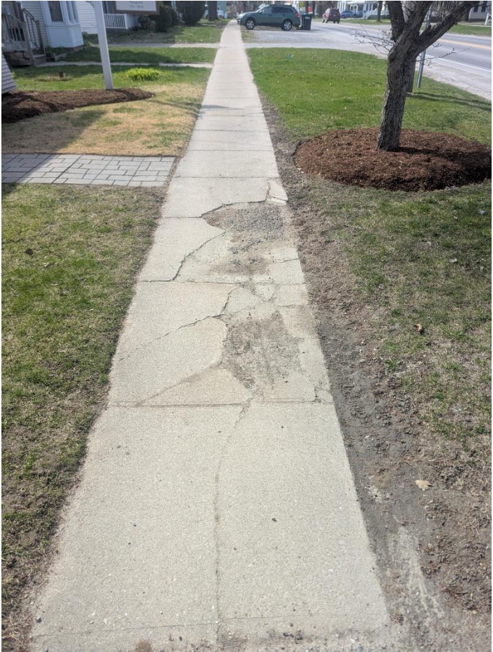
Deteriorated Concrete
