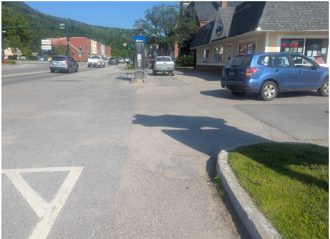
Photo 1 Gap in Sidewalk at Champlain Farms
