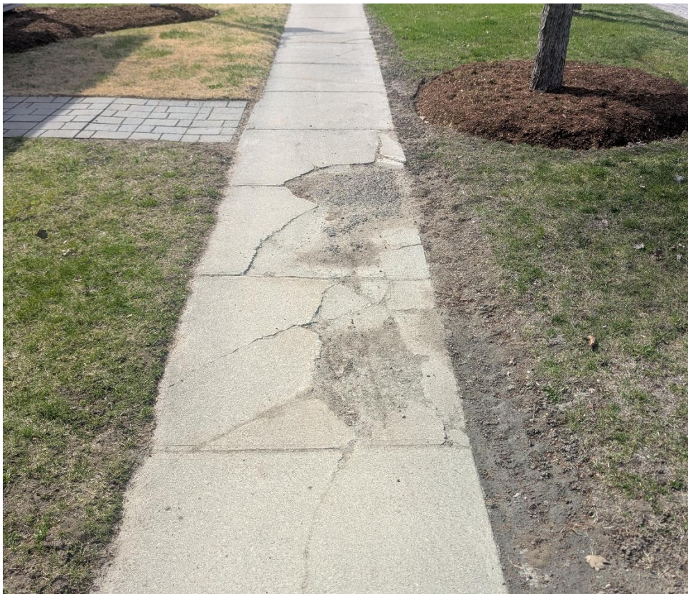
Photo 3 Damaged Concrete
