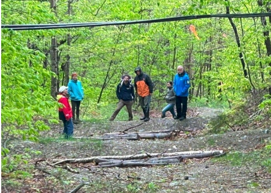
Figure 6. Broad-based dips along the Spring Road have been filled with small-diameter logs / branches to facilitate truck passage. Note overhead sap main lines. As viewed on 22 May 2025 during field site visit with Bristol Conservation Commission led by David Brynn. Photo credit: Aidan Lenihan.
