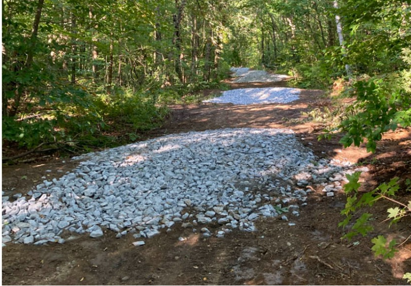
Figure 5. Seth Hill road segment of 10-12% grade, treated with broad-based dips containing 4-6" crushed stone. Photo credit: David Brynn.
