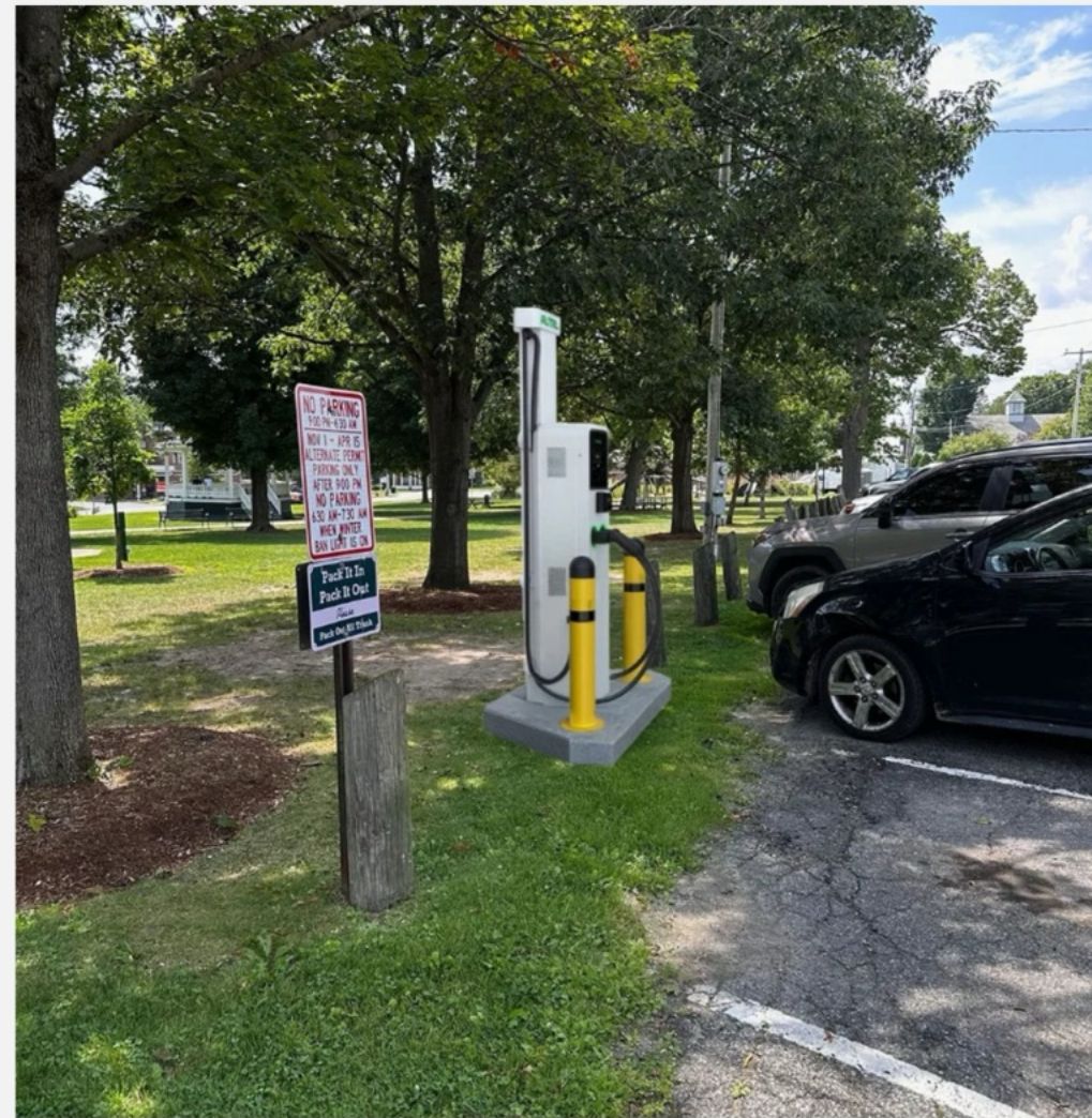
The 2-port pedestal in place
