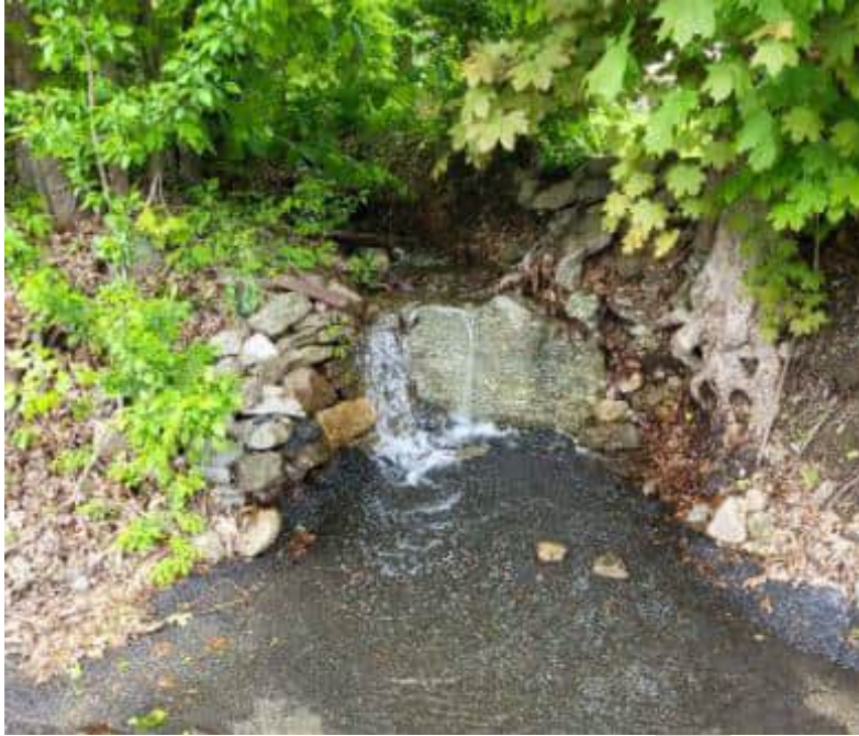
Figure 3: Flow onto the Mountain Street paved swale at the intermittent watercourse
