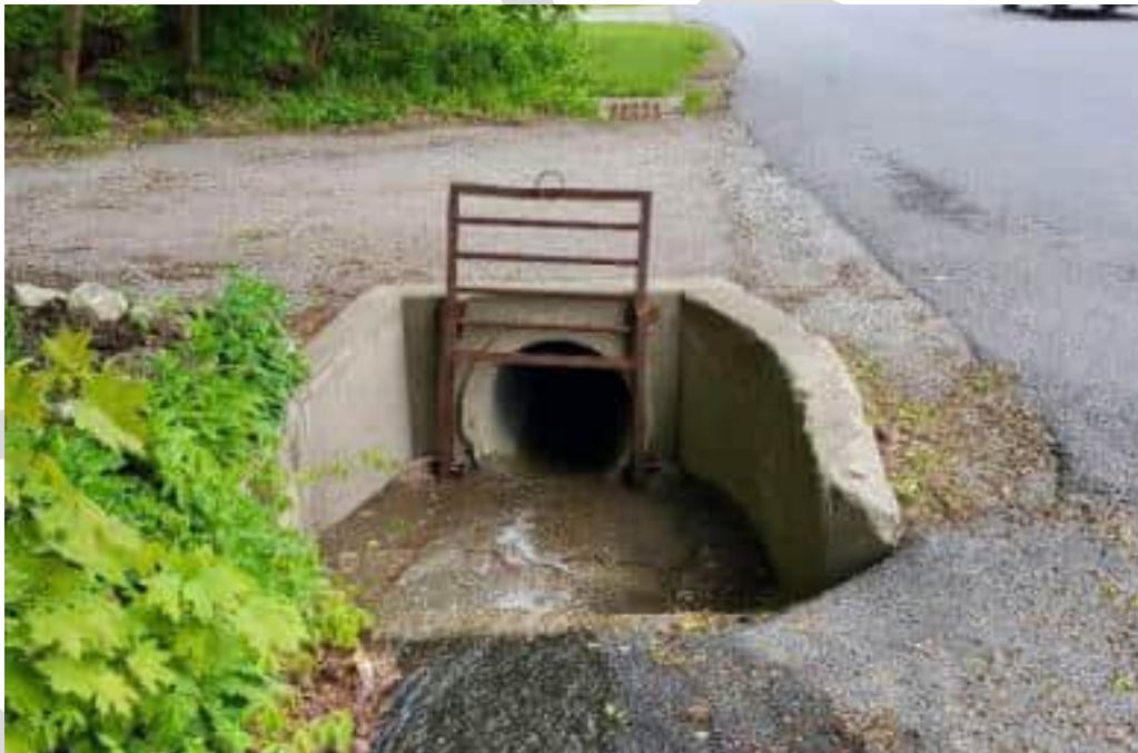
Figure 4: Three-sided Concrete headwall and trash rack at 24-inch RCP inlet to the Mountain Street enclosed drainage system
